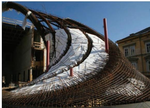
**Fig. 11** Supporting scaffold, placing of reinforcement
