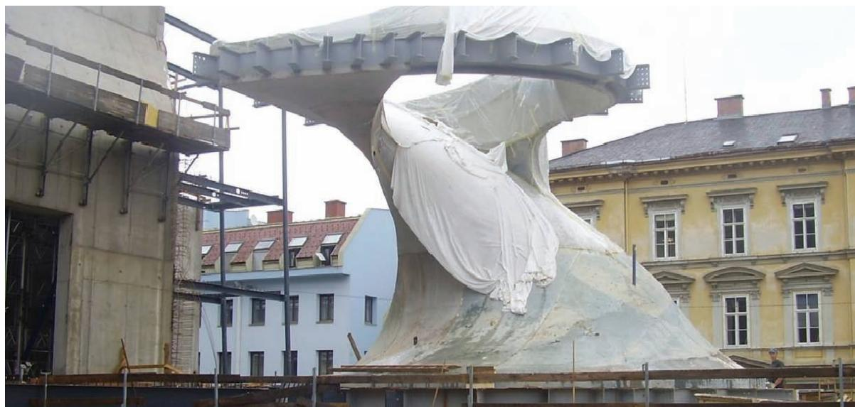
**Fig. 12** The Twist after striking
