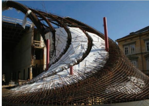
**Fig. 11** Supporting scaffold, placing of reinforcement
